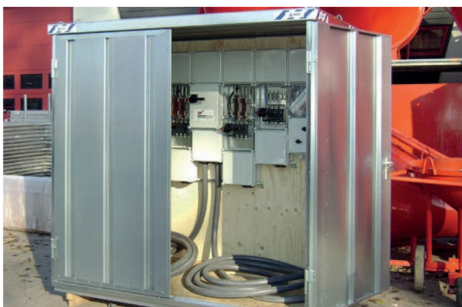
As housing for a power distribution box
