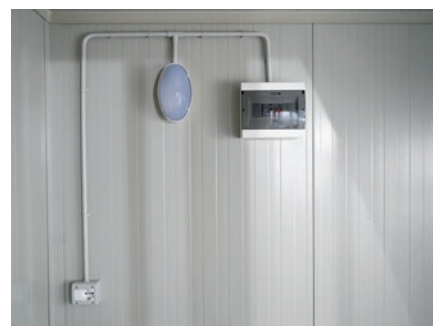
Electrical package (10W LED light with switch, 16A Schuko plug, fuse box, outdoor connection and earth cable)
